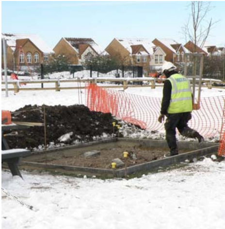
The snow didn't stop the work – picnic table platforms
